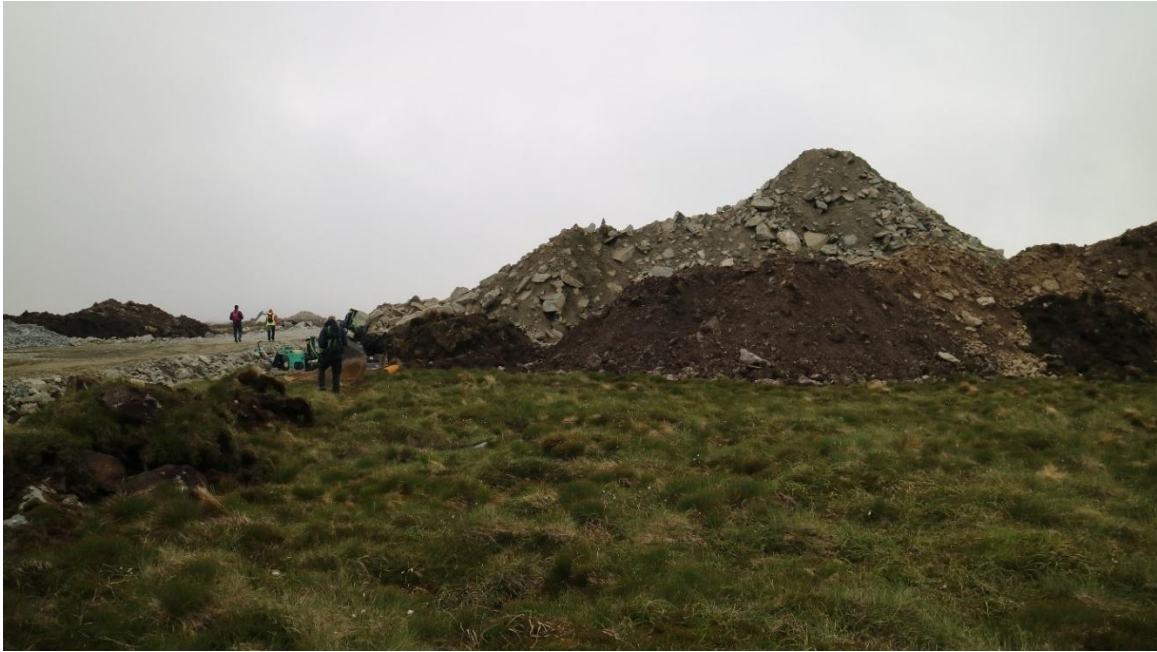
Okla wind farm, on a mountain in western Norway. Here even the Norwegian bedrock was too fractured for safely anchoring wind turbines into it, so gravity foundations had to be built. This mound shows mass excavated just to anchor one 150 m tall wind turbine.
